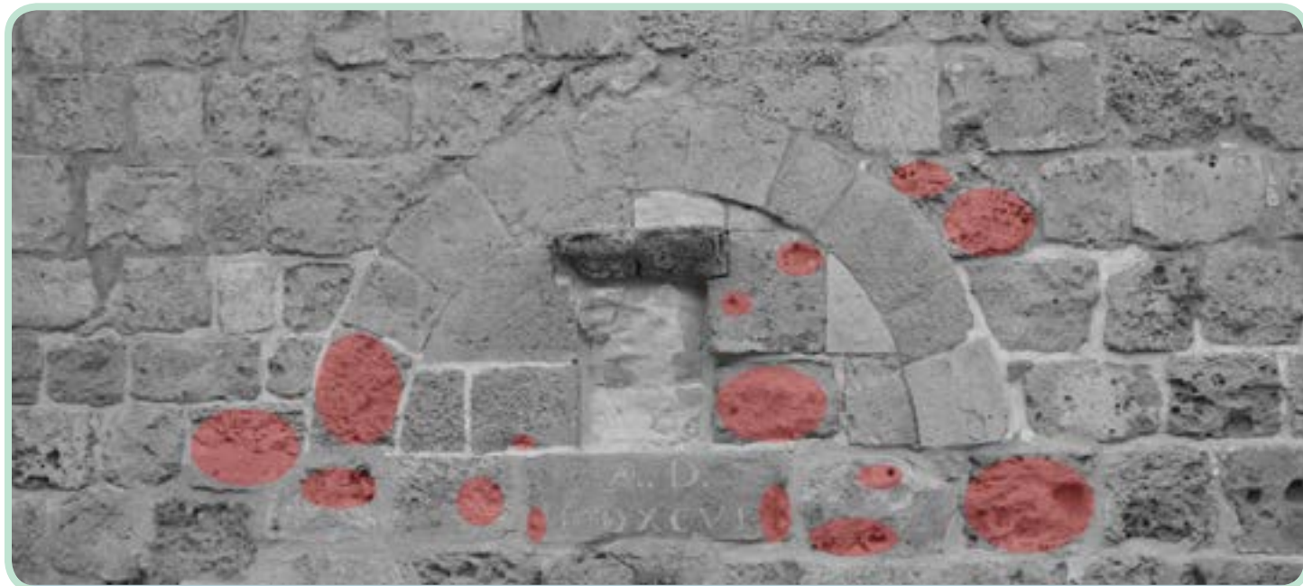
The red indicates the deteriorated sandstone
