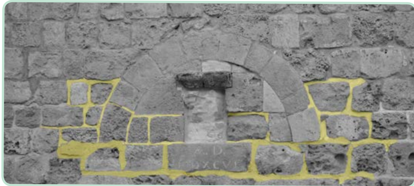
The yellow indicates where the cement should be replaced with hydraulic lime mortar with sandstone particles
